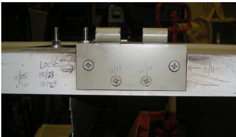
Figure 7.--Loose screws noted on one hinge during the testing.
