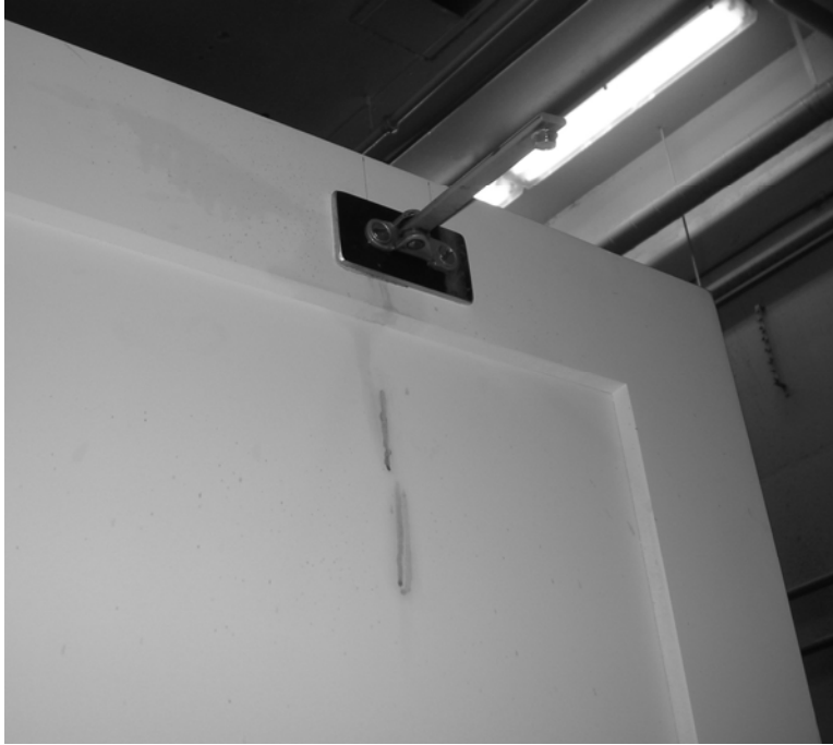
Figure 4.--Closer bar attached to door.
