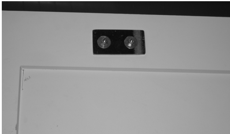
Figure 5.--Closer bar backer plate.
